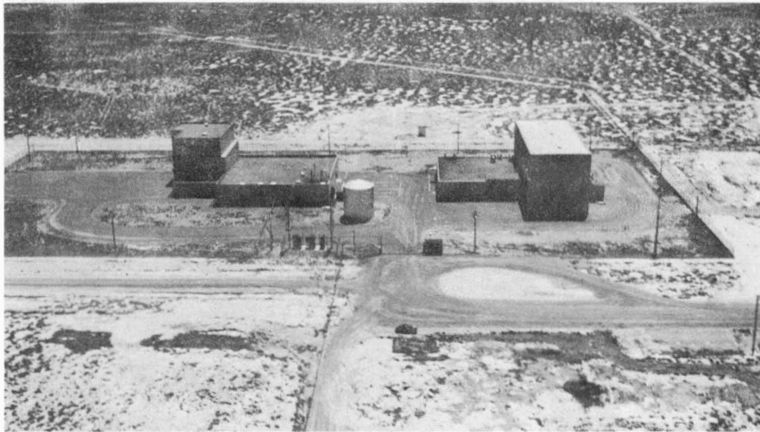
Figure A-4 - Low Power Test (LPT) and Shield Test Pool (STP) facilities. Fuel elements were inserted into the reactor in the LPT for an initial critical checkout. This was followed by low-power testing to evaluate nuclear characteristics prior to power operation. Operations were viewed by means of remotely operated television. (U-3343-55)
