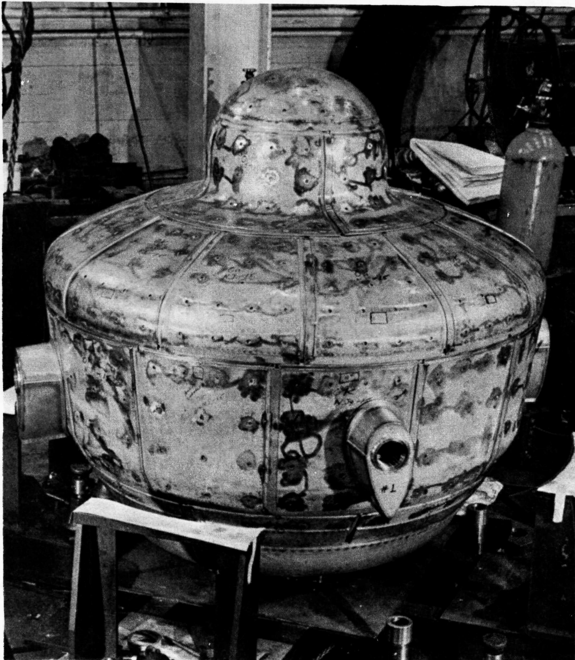
Fig. 5.38 – Insulated rear shield plug island (Neg. U36136C)
