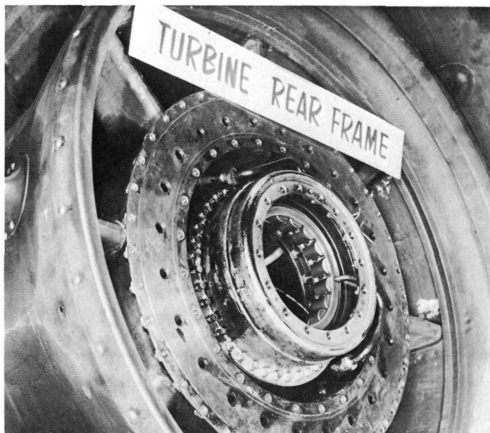
Fig. 6.23 - Turbine rear frame assembly (Neg. 245558)
