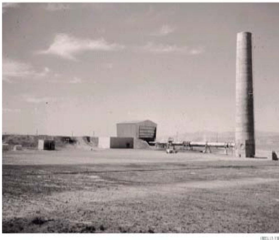
Figure 2-4 150-foot Exhaust Stack
