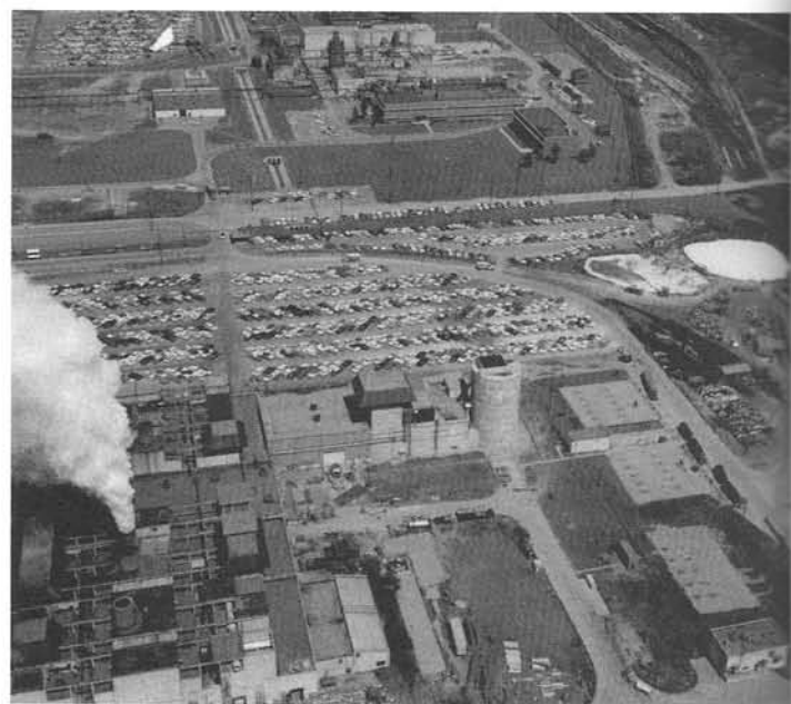
Above: The General Electric Evandale Ohio Plant. Built by Curtis Wright A/C Company during WWII. Photo Circa 1955. It was at this plant that all nuclear engines were designed and tested with chemical fuels only. All "Hot" testing was done at the Idaho Test Site.
