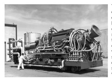
Their purpose was solely to demonstrate feasibility of Weighing design. over hundred thousand pounds, each, they were built on railcars to facilitate movement to remote test locations. After each test, the reactor's railcar would be returned to a heavily shielded maintenance bay for disassembly & analysis. Their size can best be appreciated when viewing this photo.
